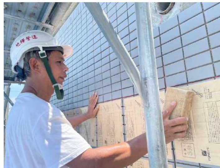
R3F外牆磁磚施作
