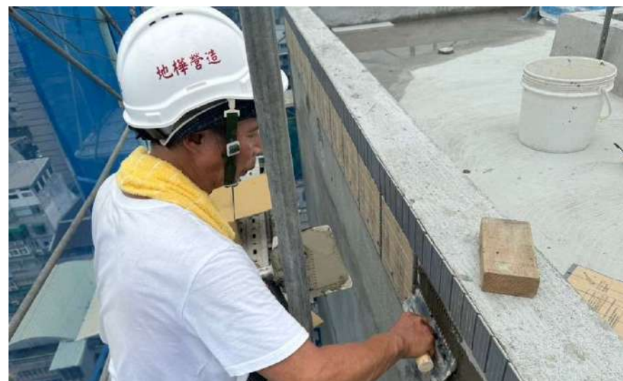
R3F外牆磁磚施作
