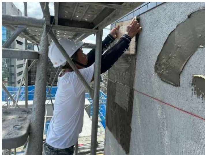
R3F外牆磁磚施作
